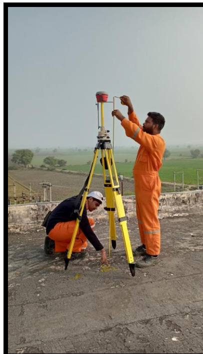
Topographic survey in progress
